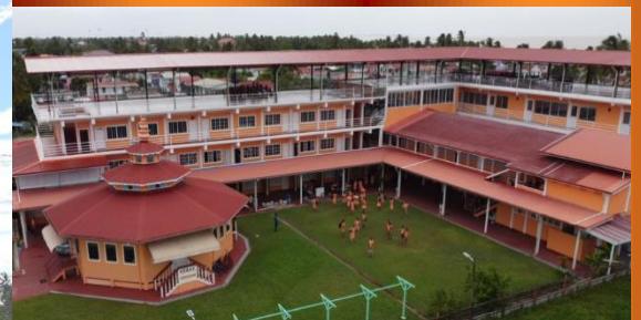
The final structure connecting the three buildings and the newly renovated terrace in 2021
