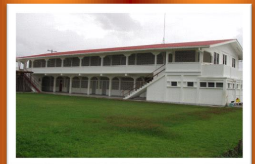
The “new building” in which classes began in September 2002.
